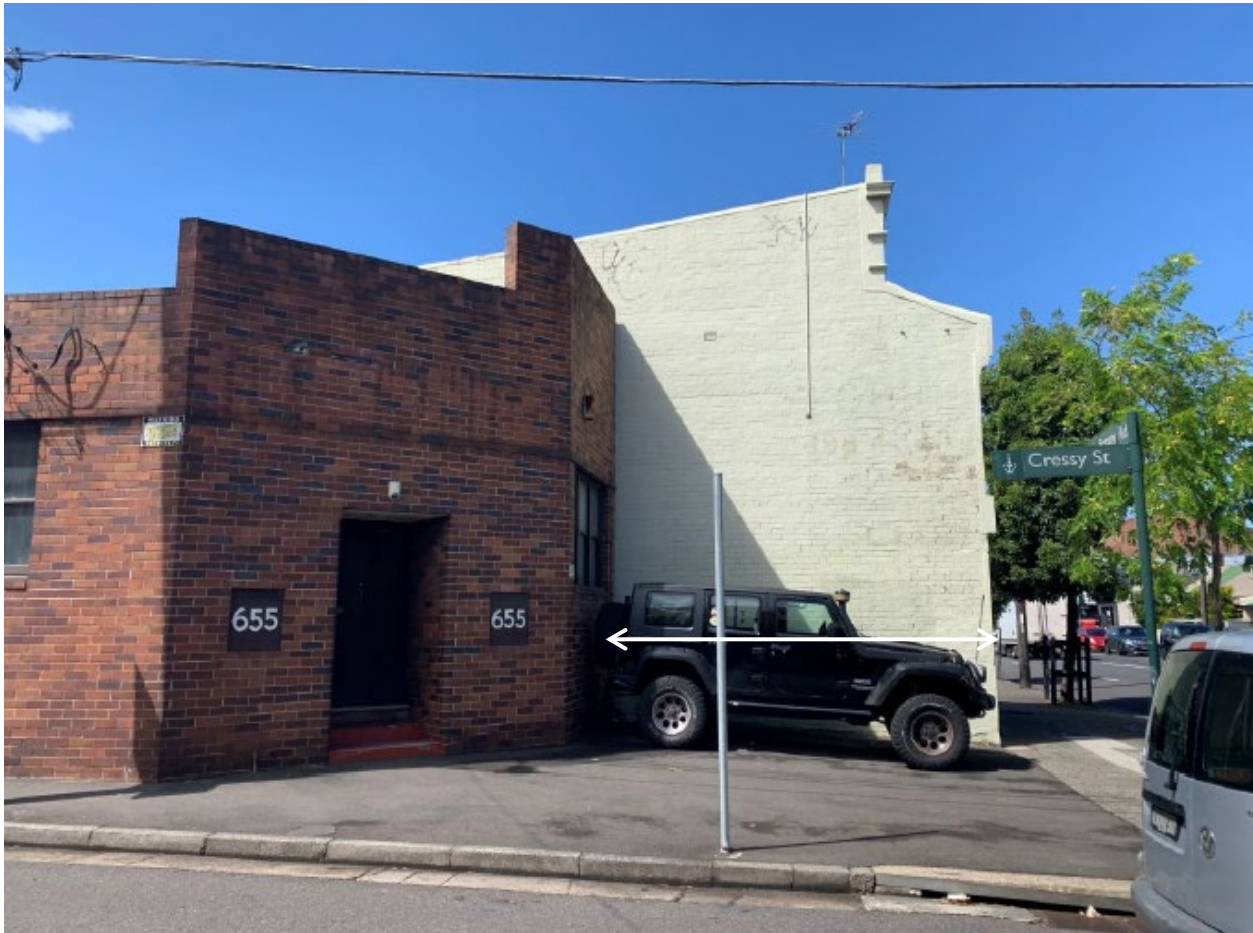
north elevation of existing terrace viewed from Cressy Street
